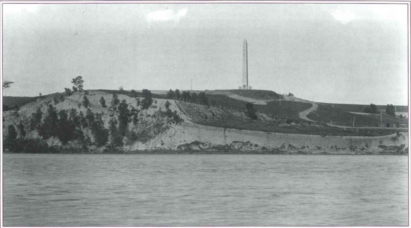
The view of the monument from the Nebraska side of the Missouri River. The monument stands out prominently for many miles on the prairie.
